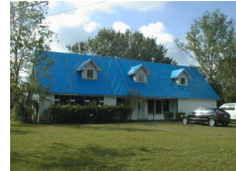
FEMA Temporary Roof Installation
